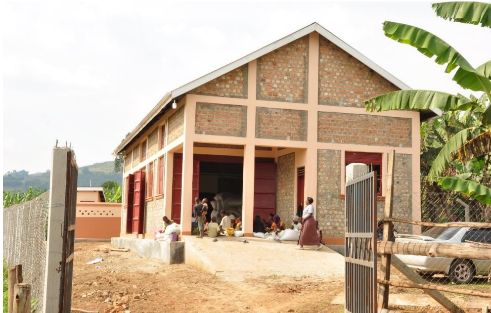
Karubanda Tukorerehamwe Cluster bean storage facility, Rukiga district
