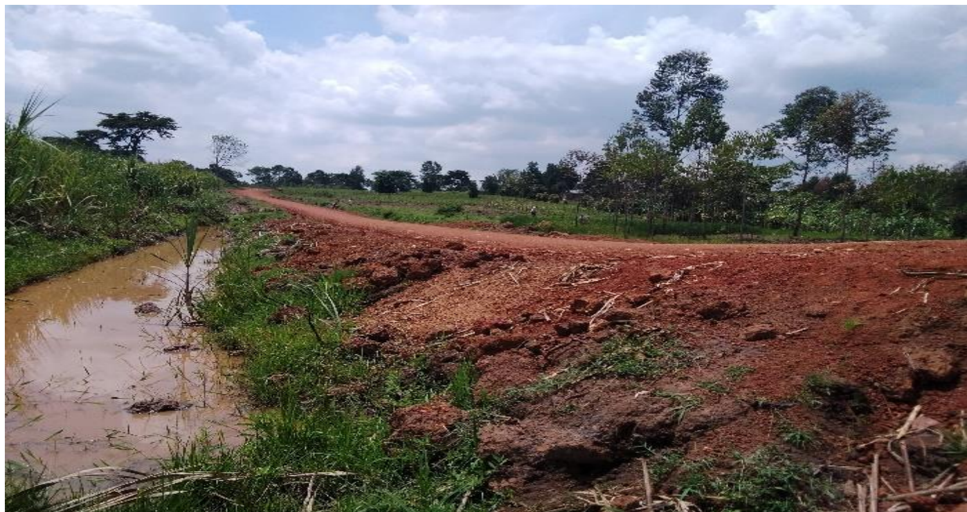
Part of the swamp sections filled in at Butende- Ibulanku- Buyede- Idudi Road- Iganga district
