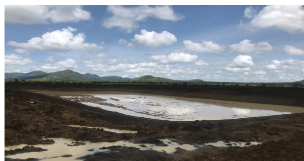
Omunga Valley Tank under construction in Abim District
