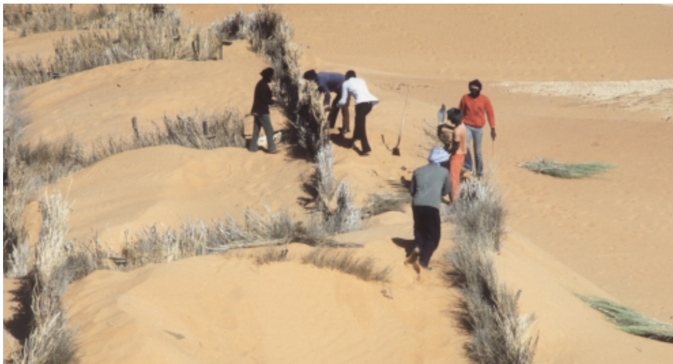
Dune fixation with windbreak fences, Mauritania
