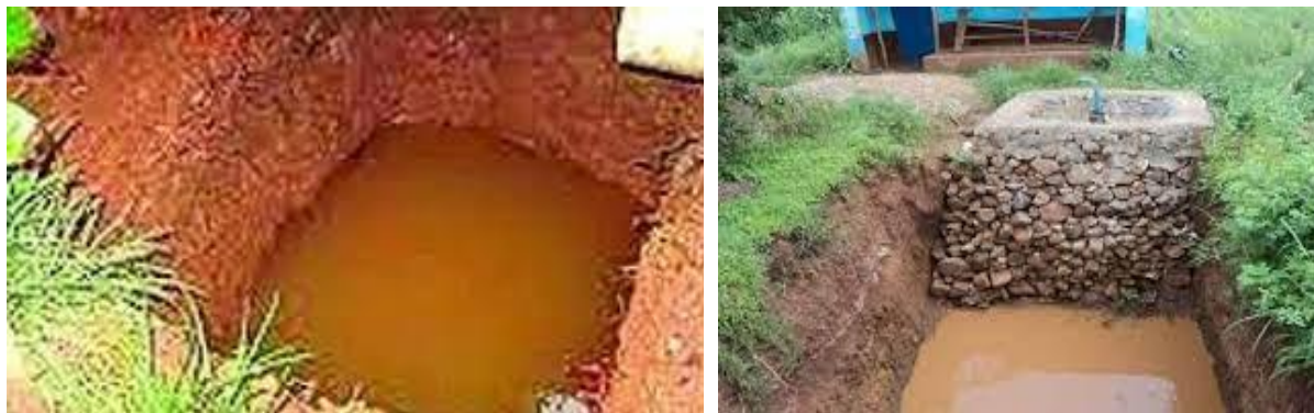
Figure 13: Pond water harvesting structure for irrigation
